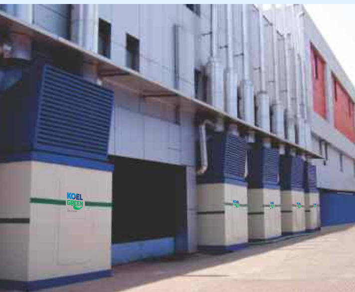
SHOPPING MALLS 5 X 500 kVA Typical installation
