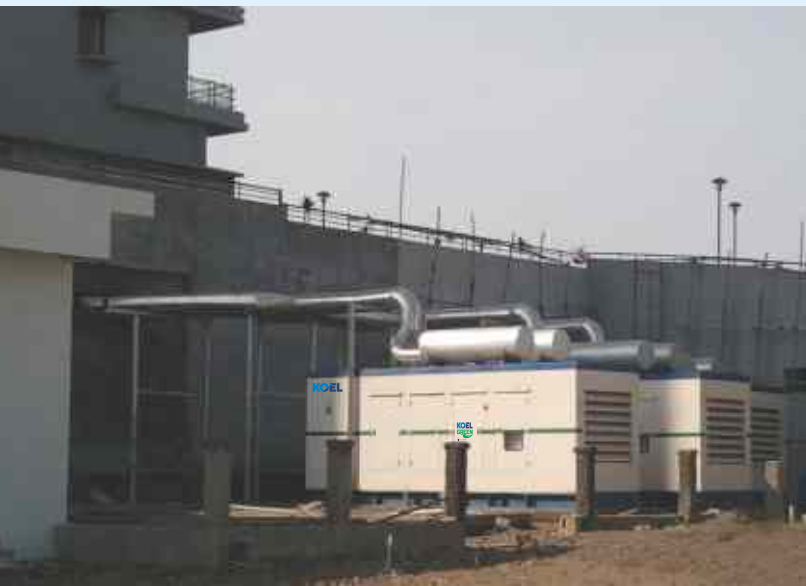
HIGH RISE APARTMENT COMPLEX Extensive exhaust piping
